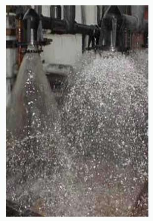
• HCCT cooling tower distribution system consists of gravity distribution with large orifice nozzle, which greatly reduces clogging and assure constant performance capacity between maintenance intervals. When nozzle cleaning is required, each nozzle can be easily removed in place and cleaned.
